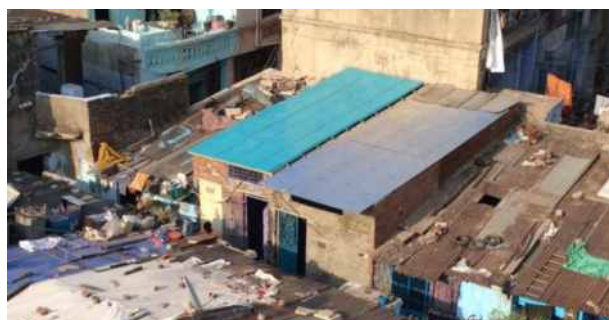
Mod-Roof, A modular roof system that offers better weather protection and insulation and brings down indoor temperatures by 5 to 6 degree Celsius.
